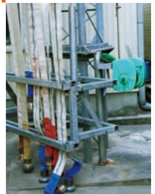
For drying a fire-fighting hose
